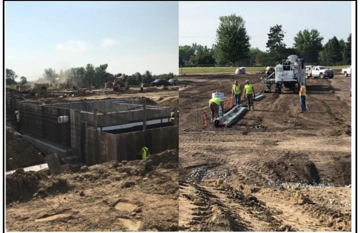
CLCC: installing foundation walls.
